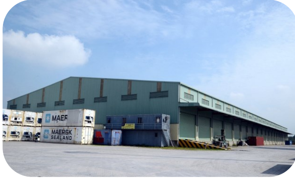
CFS & BONDED WAREHOUSE
